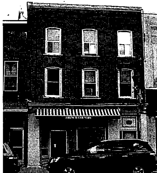
32. Retractable awning does not obscure architectural detail, such as the storefront cornice at 255/257 Main Street (Source: ERA Architects)
