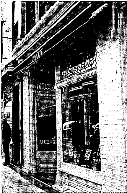
28. Example of an existing and well-maintained historic storefront at 255/257 Main Street (Source: ERA Architects)
