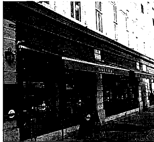
31. Retractable awning (Source: City of Kingston)
